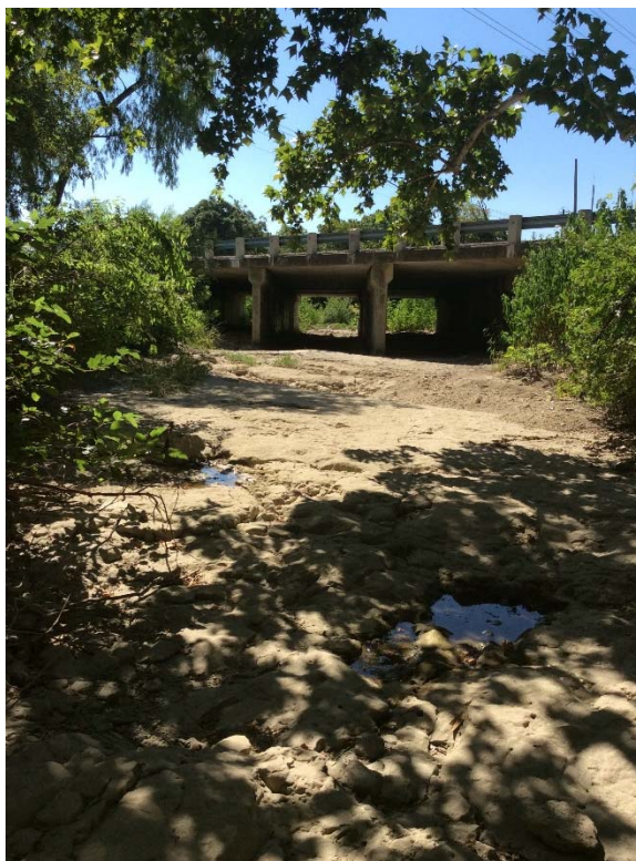
Photograph 21: Williamson Creek (S-6) upstream of US 290/SH 71 crossing; facing south.
