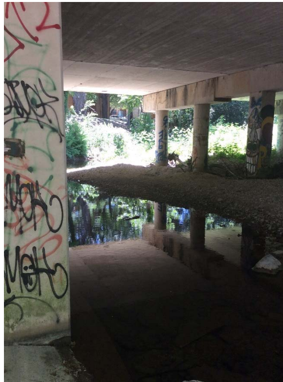
Photograph 16: S-5 under SH 71 looking west
