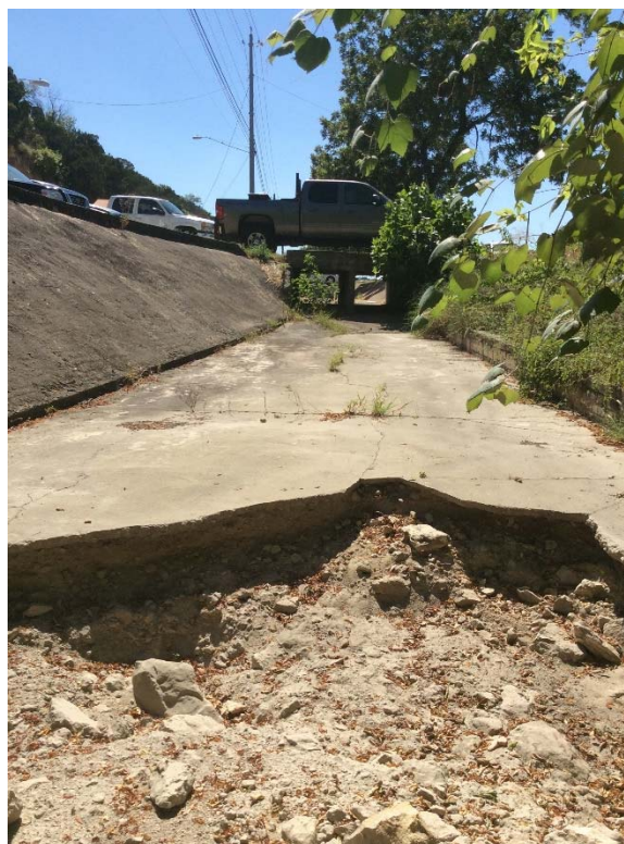
Photograph 24: Unnamed tributary to Williamson Creek (S-7) south of US 290/SH 71; facing east.
