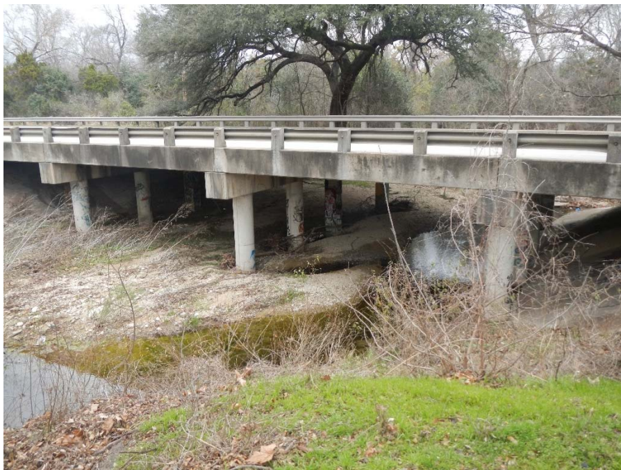
Photograph 20: Williamson Creek at SH 71 bridge; facing northeast.
