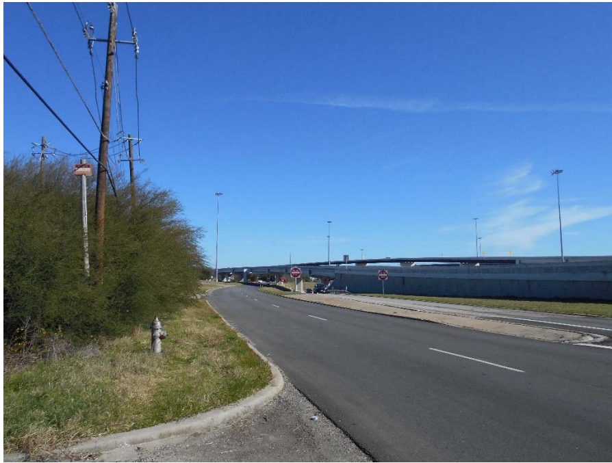
Photograph 17: Native invasive vegetation and Urban Low Intensity along US290/SH71 at William Cannon; facing east.
