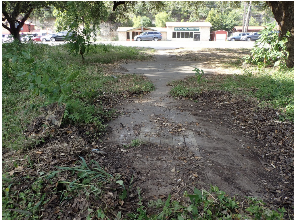
Figure 10. Concrete and brick improvements near Oak Hill marker. Facing south.
