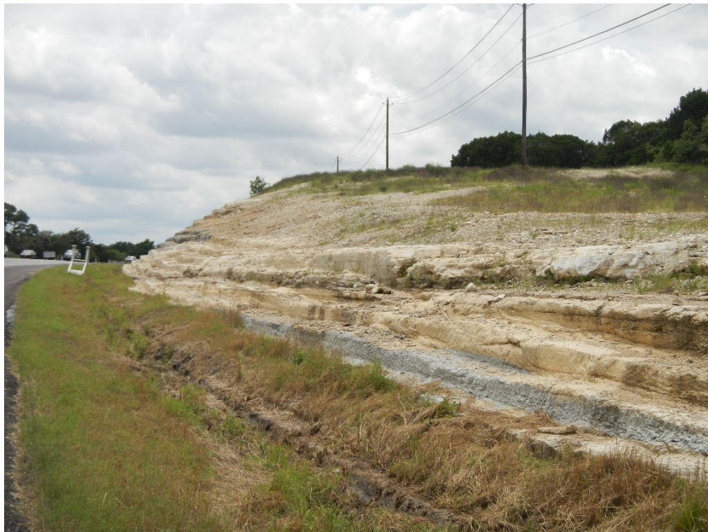
Figure 12. View of exposed bedrock visible in road cut below grade and into bedrock. Facing northwest.
