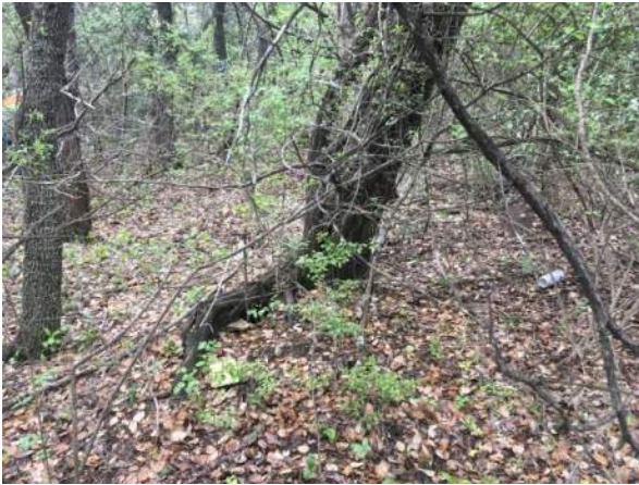
Feature F-10 – Hole (possibly and animal hole) at the base of a tree. Located within the existing right-of-way south of US290 and east of RM 1826.
