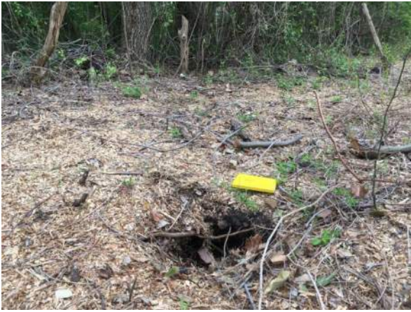
Feature F-7 – Cavity located north of the existing US 290 right-of-way along the transmission line corridor.
