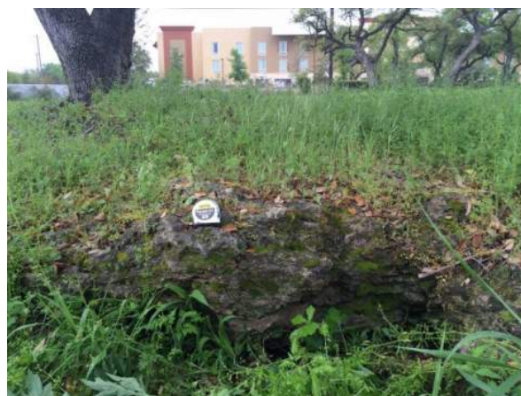
Feature F-2 solution cavity situated along the base of a bedding outcrop
