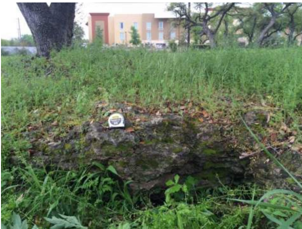
Feature F-4. Zone of fractures located south of US290 along the southern margin of the TxDOT right-of-way
