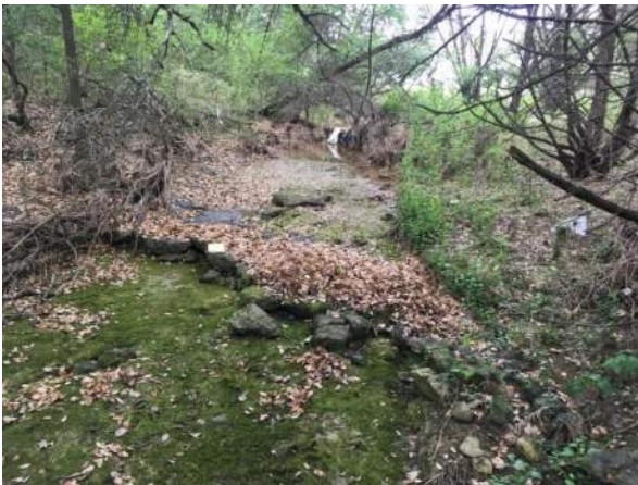
Feature F-12 – A solution enlarged fracture in a streambed. Feature F-12 is located within existing right-of-way south of US290 and east of RM 1826.
