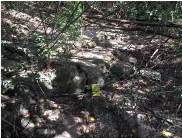
Feature F-8 – Area of fractures located south of the intersection of Old Bee Caves Road and the Bell Hill Country Apartments entrance road. On proposed right-of-way.
