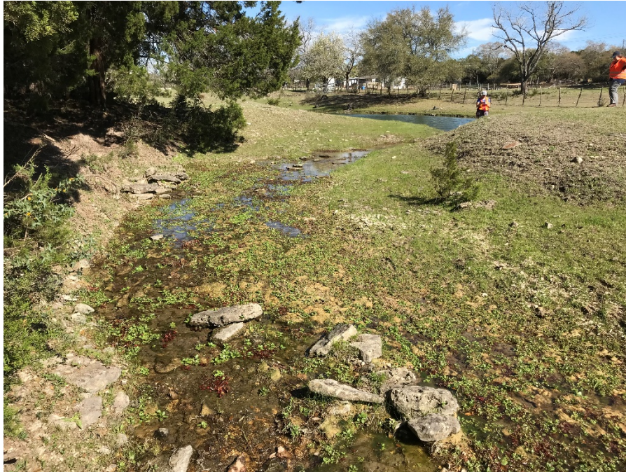
Photograph 37: Unnamed tributary to Williamson Creek (S-11) within SH 71 detention pond site; facing north.
