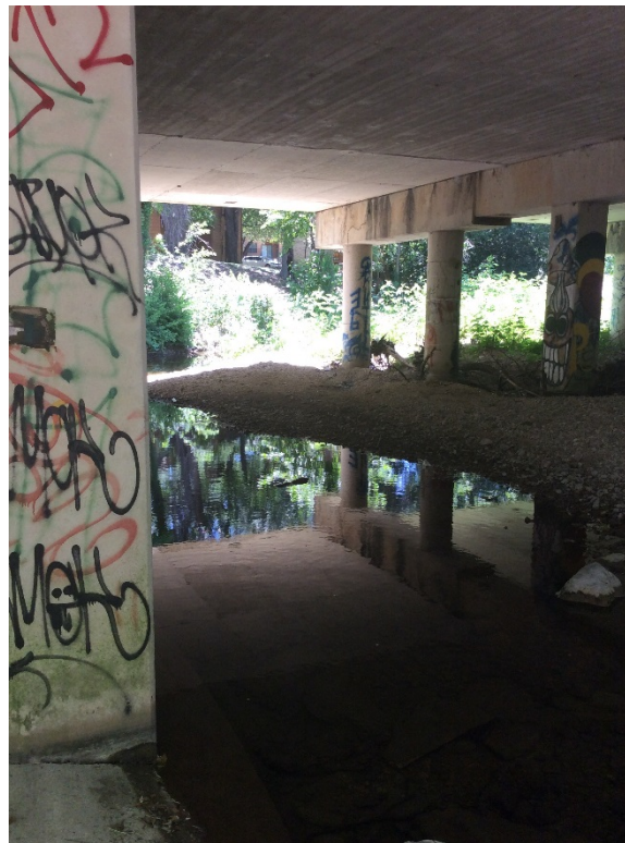
Photograph 24: S-5 under SH 71 looking west
