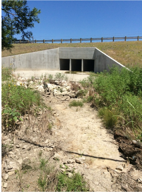
Photograph 21: Wheeler Branch (S-3) south of 290; facing north.
