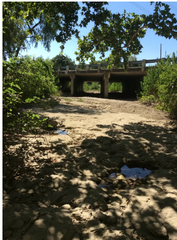
Photograph 30: Williamson Creek (S-6) upstream of US 290/SH 71 crossing; facing south.
