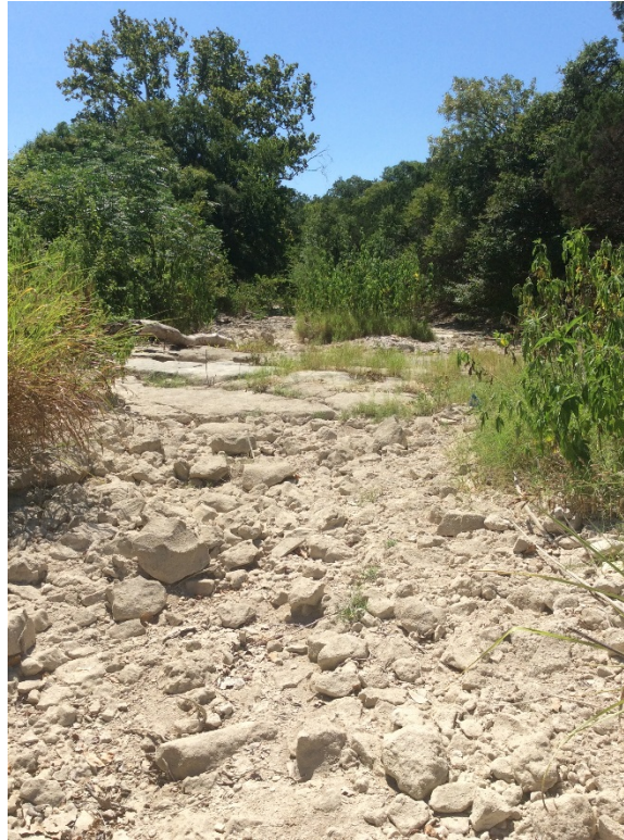
Photograph 31: Downstream of US 290/SH 71 crossing of Williamson Creek (S-6); facing south.
