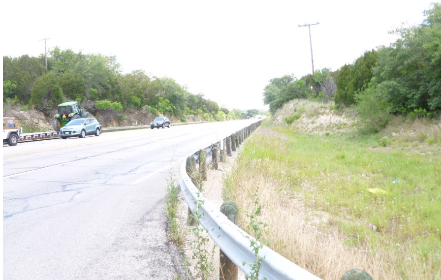
Photograph 5: Oak-juniper woodland and native-invasive vegetation along US 290; facing west.
