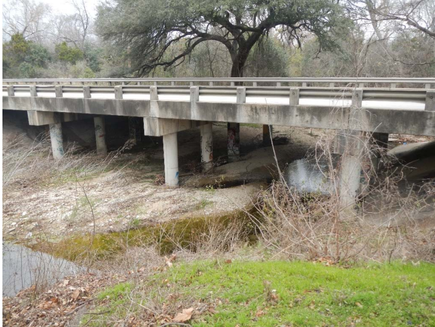
Photograph 17: Williamson Creek at SH 71 bridge; facing northeast.
