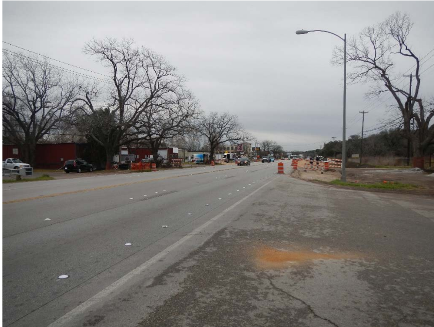
Photograph 1: Commercial land use along SH 71 south of Williamson Creek crossing; facing south.
