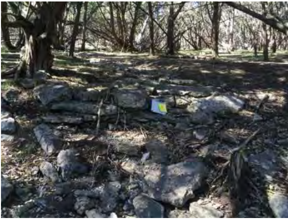
Feature F-9 – Area of fractures located within proposed right-of-way for the detention pond on the southwest side of SH 71.
