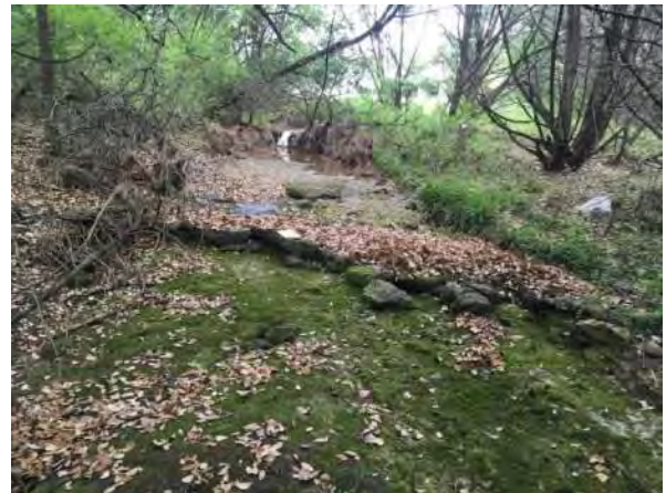
Feature F-12 – A solution enlarged fracture in a streambed. Feature F-12 is located within existing right-of-way south of US 290 and east of RM 1826.
