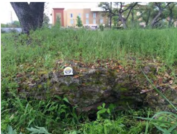
Feature F-4. Zone of fractures located south of US 290 along the southern margin of the TxDOT right-of-way
