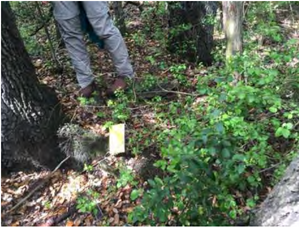
Feature F-11 – Enlarged fracture, which consisted of a rock bench with a weaker area underneath. This feature was located south of US 290 and east of RM 1826.
