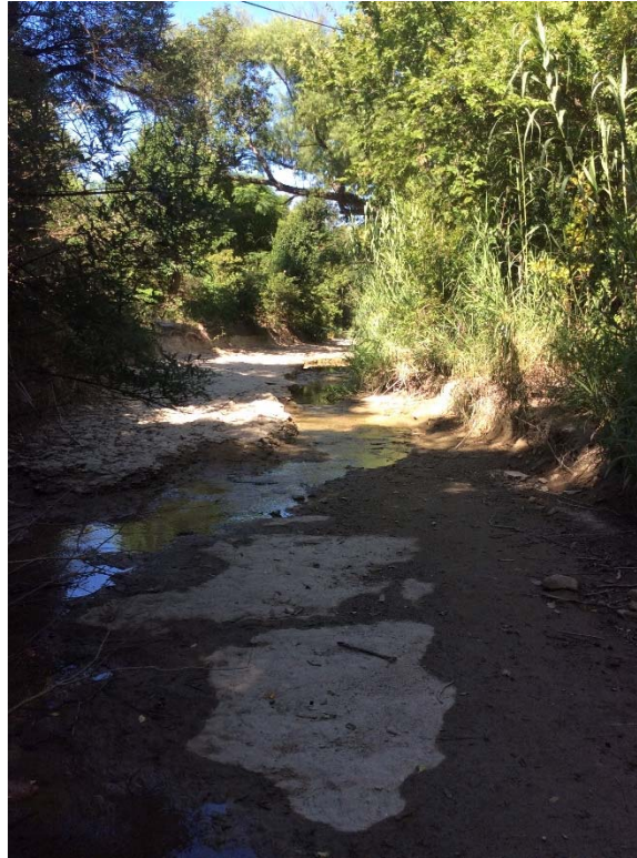
Photograph 23: Along Williamson Creek (S-6) north of US 290/SH 71; facing east.
