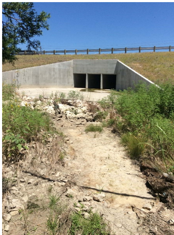
Photograph 18: Wheeler Branch (S-3) south of 290; facing north.
