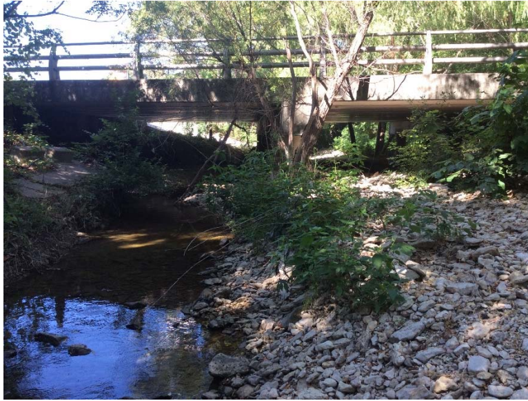
Photograph 29: Williamson Creek (S-6) at William Cannon Road crossing; facing east.
