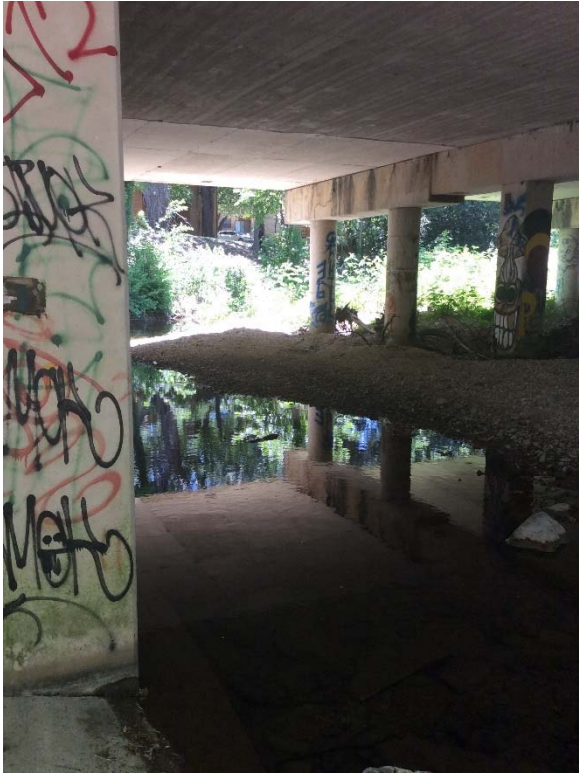
Photograph 21: S-5 under SH 71 looking west
