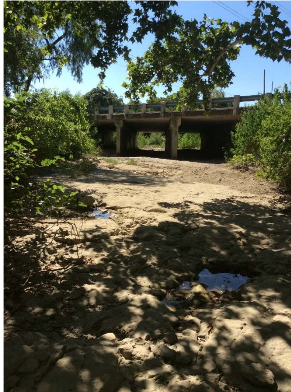
Photograph 27: Williamson Creek (S-6) upstream of US 290/SH 71 crossing; facing south.
