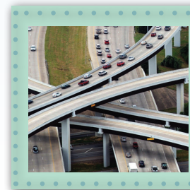
Freeway Interchange $325 million
