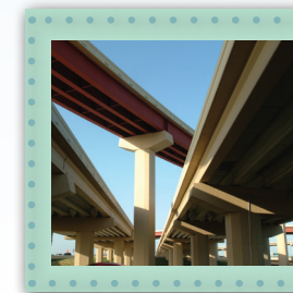
Overpass $6.8 million per lane mile
