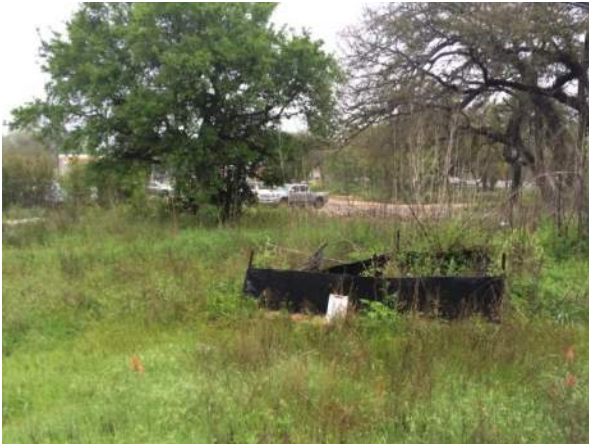
Feature F-6 – solution cavity located along the southern limits of the TxDOT right-of-way south of US290
